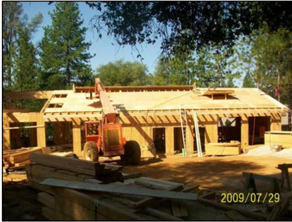
Building "E" framing in progress
