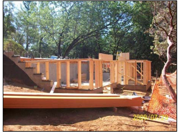
Building "B" basement walls framing in progress
